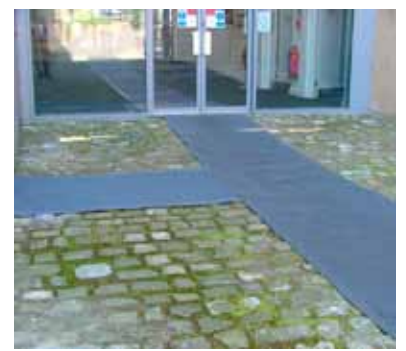
FRONTRUNNER XT CREATES A SAFE EXTERIOR WALKWAY ON SLIPPERY COBBLES AT THE UNIVERSITY OF GREENWICH
