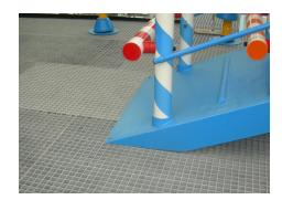
"This project was particularly interesting because of the inherent difficulty with the structural design of the floor – the twin problems of how to deal with a lot of water, as well as to provide a safe and comfortable surface on which small children could play. Now, the water flows away easily, maintenance is eliminated and, of course, management, parents and children are all very happy!"
