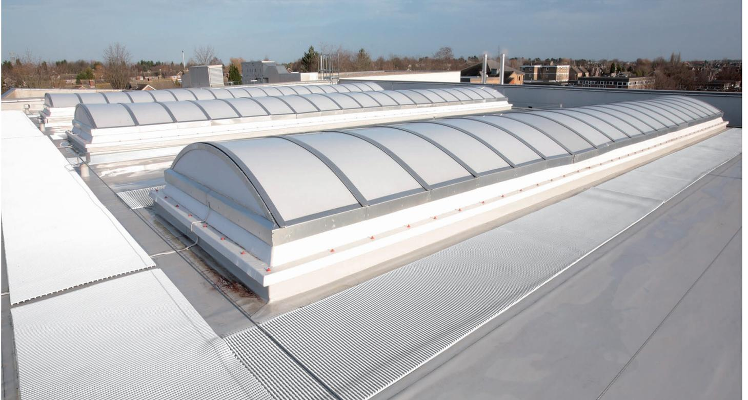
**Crossgrip TPO has been specifically created to protect flat roofs from heavy foot traffic, dropped tools and maintenance equipment.**
