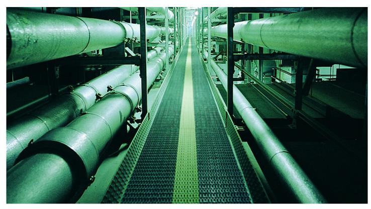
Certified slip resistant with a light-emitting band running down the centre, Heronair Photoluminescent glows in the dark, making it the perfect matting to mark escape routes along walkways in case of lighting failure.
